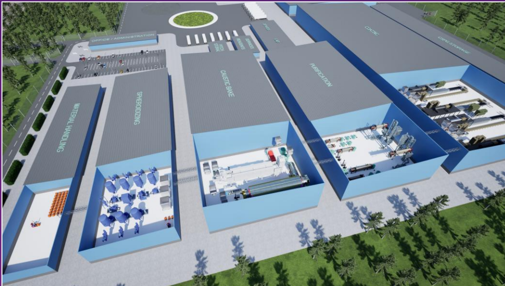
Figure 7: Milling, Shaping, Purification, Coating and Packaging stages within the refinery
